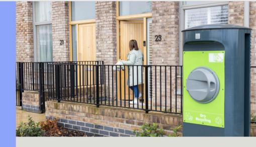
The Envac waste collection system utilises vacuum suction to remove household waste. This system reduces air pollution and has quadrupled household recycling rates beyond comparable averages.
